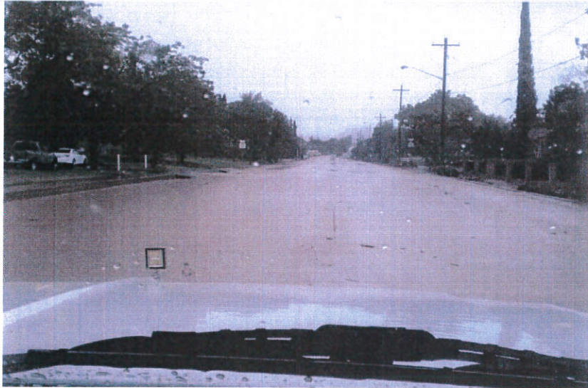
Figure 2a – Main Street Flooding.
