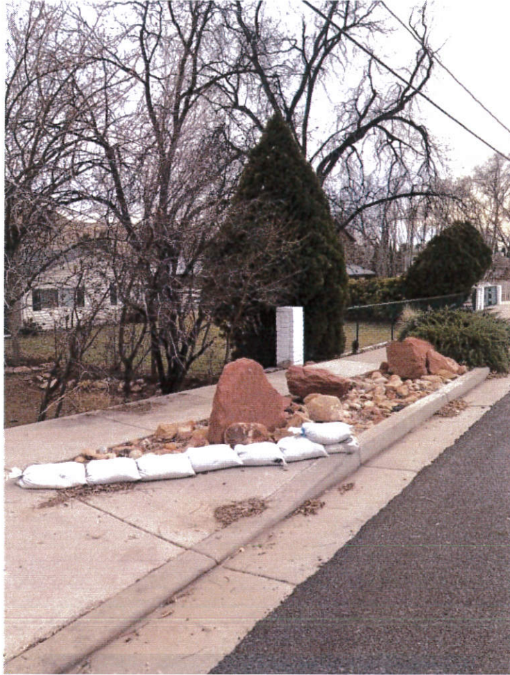
Figure 2c- Sand Bags to Prevent Overtopping of Water
