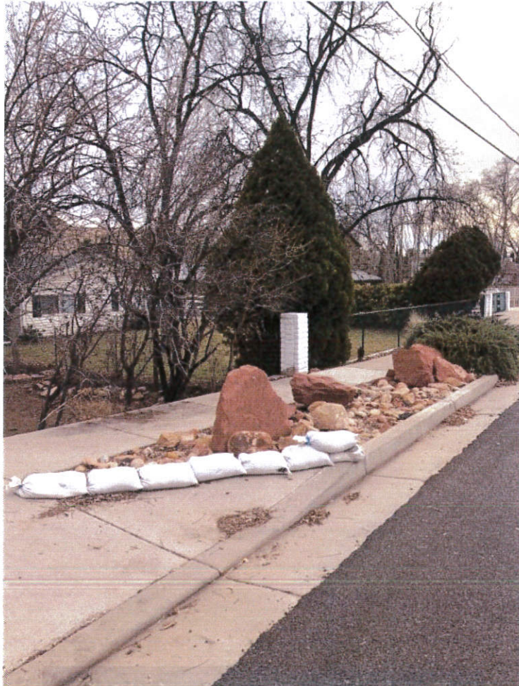
Figure 2c- Sand Bags to Prevent Overtopping of Water
