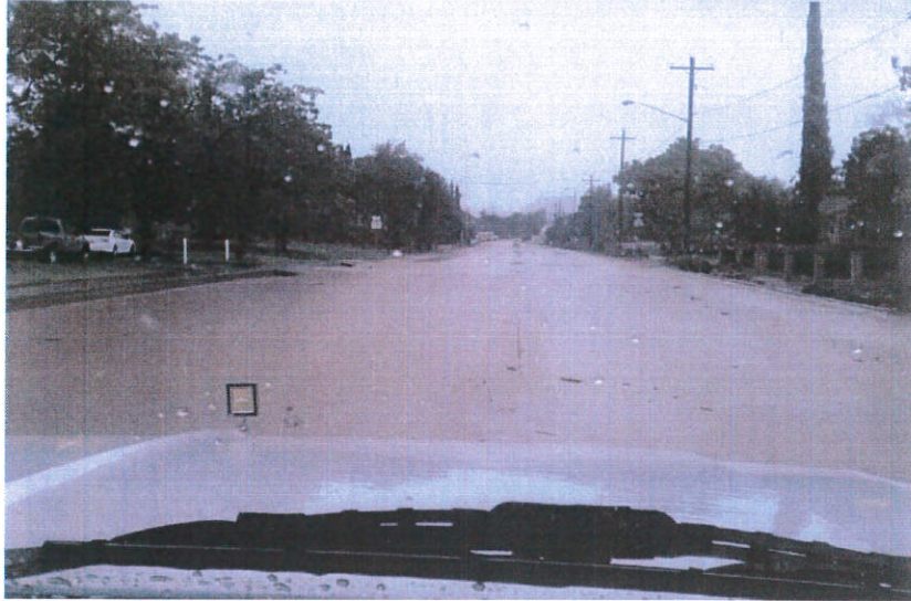
Figure 2a – Main Street Flooding.
